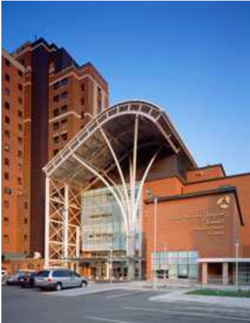
Toronto Western Hospital
